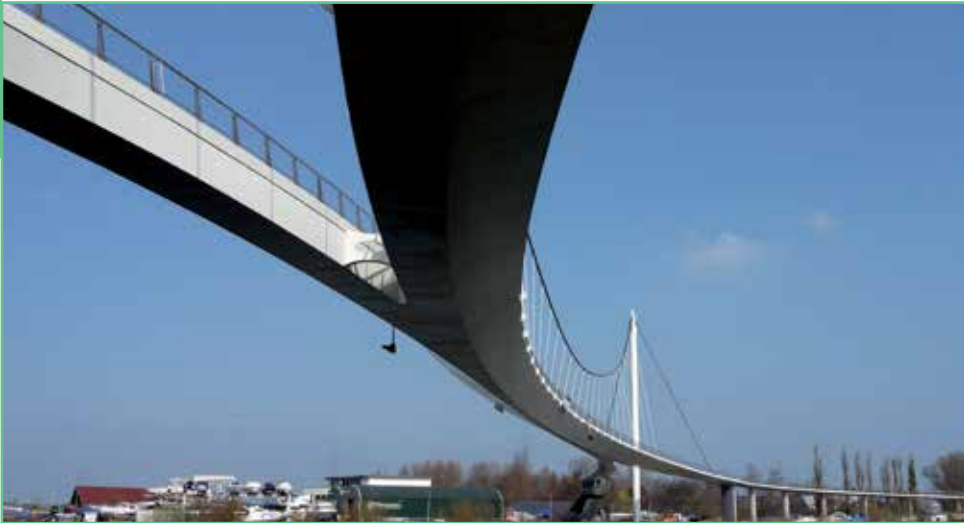
A spectacular example of the recent extension to the cycle network is the Nescio bridge, which rises 11 metres above the Amsterdam-Rhine canal to allow ships to pass below it. With a total length of 780 metres and a 1:40 slope, the construction ensures a comfortable climb for cyclists.
